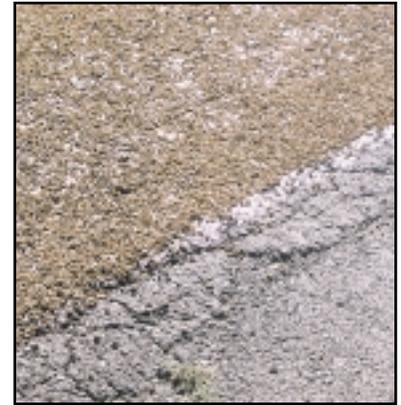
A thin application of LWA shows oil around the particles next to the exposed edge of the old deteriorated road surface.
